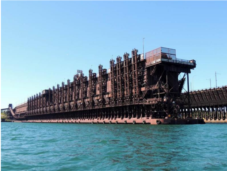
Caption: The Duluth Ore Dock – one of the longest iron ore dock in the world
