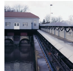
Open the gates! Cable trolley system program 0330 on a lock
